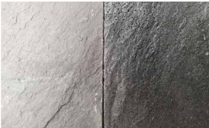
A1 panel directly after demoulding.
