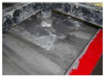
3 layers of A1 Triaxial fibre is laminated on the brackets to get a strong connection.
