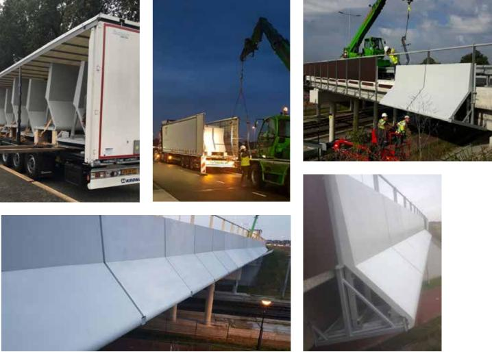
The final result is a bridge edge built up from elements that are accurately aligned. A concrete look is realized by using A1 that has 80% less weight than a bridge edge that would be made of concrete.
