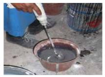
Mix the materials for the gelcoat layer: 50 parts zinc : 100 parts A1 (pbw).
