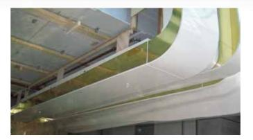
For the dilatation gap between two elements that are in line with each other in first instance it was designed to realize this by means of a joggle. However, this would involve additional inserts in each mould. Moreover, to obtain a situation that is nicely flush from one element to the other would become difficult. And there would be the risk of damaging the joggle during mounting of the element
