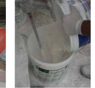
Weighing and mixing A1 Liquid, A1 Powder, Thix A and sand for the top layer.
