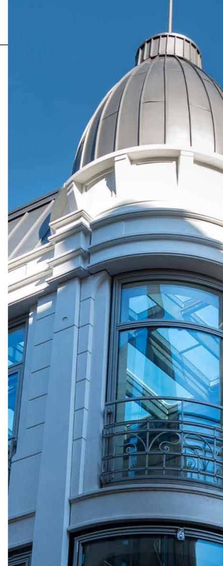
In the reconstruction of this building original materials could not be used for the reconstruction. Winhof Architects and van Wijnen Heerhugowaard choose to work with replica's made of the sustainable glass fibre reinforced and water-based system A1 (Acrylic One) material. Nedcam provides the engineering, mould making, as well as the finished façade elements.
