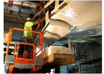
Unique moulds of milled EPS are smoothed, covered with a (red) coating system and boxed with the use of plates. After production of the A1 elements, the moulds are used for safe transportation of the A1 elements.
