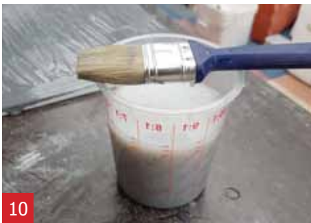
Clean the brush directly after applying the first layer.
