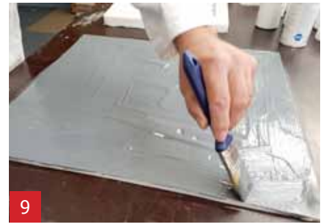
The surface must reach a thickness of 1 to 2 mm. Curing time of A1 is \pm 20 minutes.
