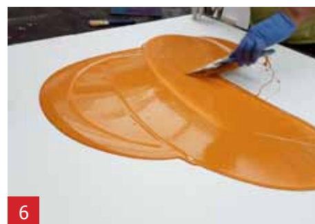
6 Apply a thin layer of A1 on the EPS with a spatula.
