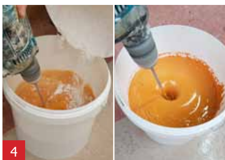
4 Then add the A1 powder to the A1 liquid and stir for 1 minut until you have a smooth surface.
