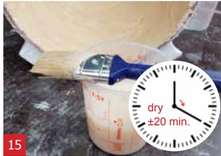
Clean the brush directly after applying the 2nd layer and again let the panel dry for  $\pm 20$  min.
